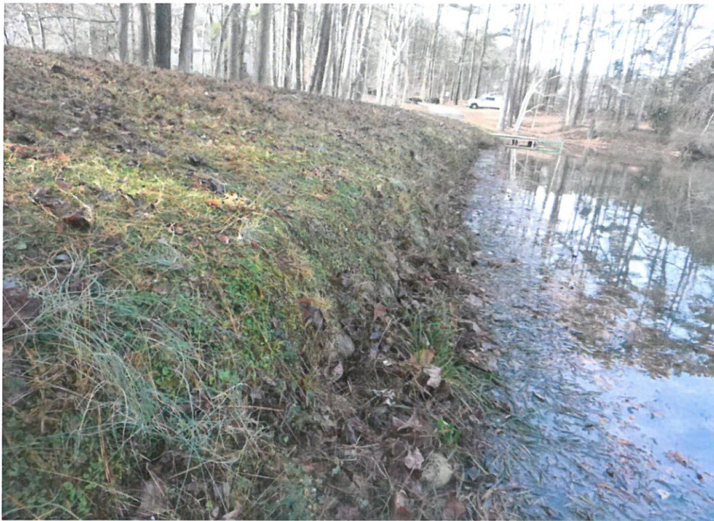
28" NEAR VERTICAL FACE ON UPSTREAM SLOPE.
