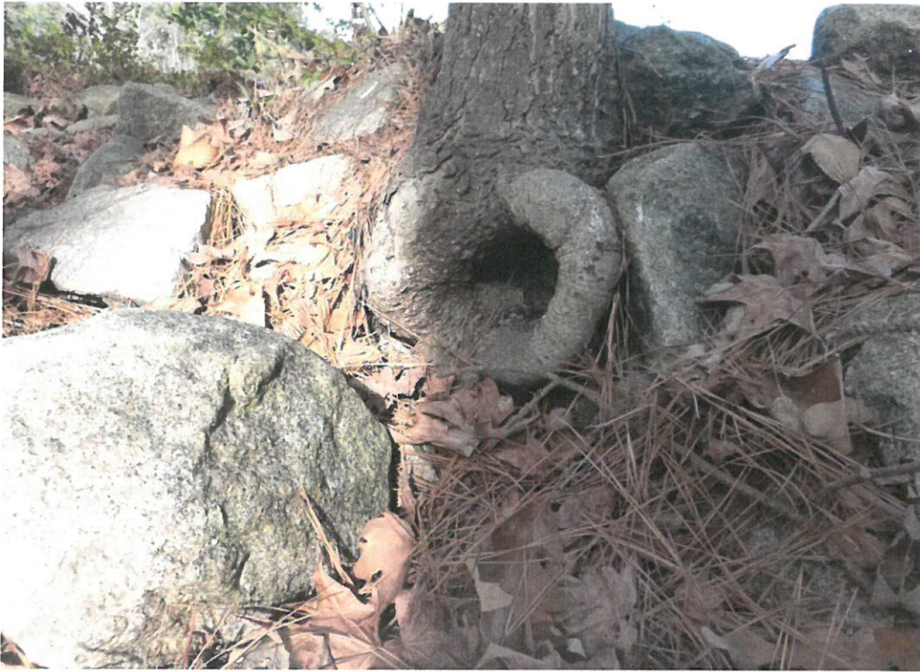
ANIMAL BURROW ALONG DOWNSTREAM SLOPE.
