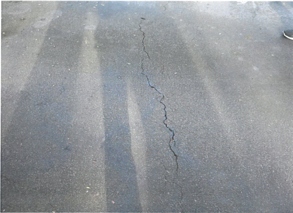
FULL WIDTH TRANSVERSE CRACK UP TO 1/4".
