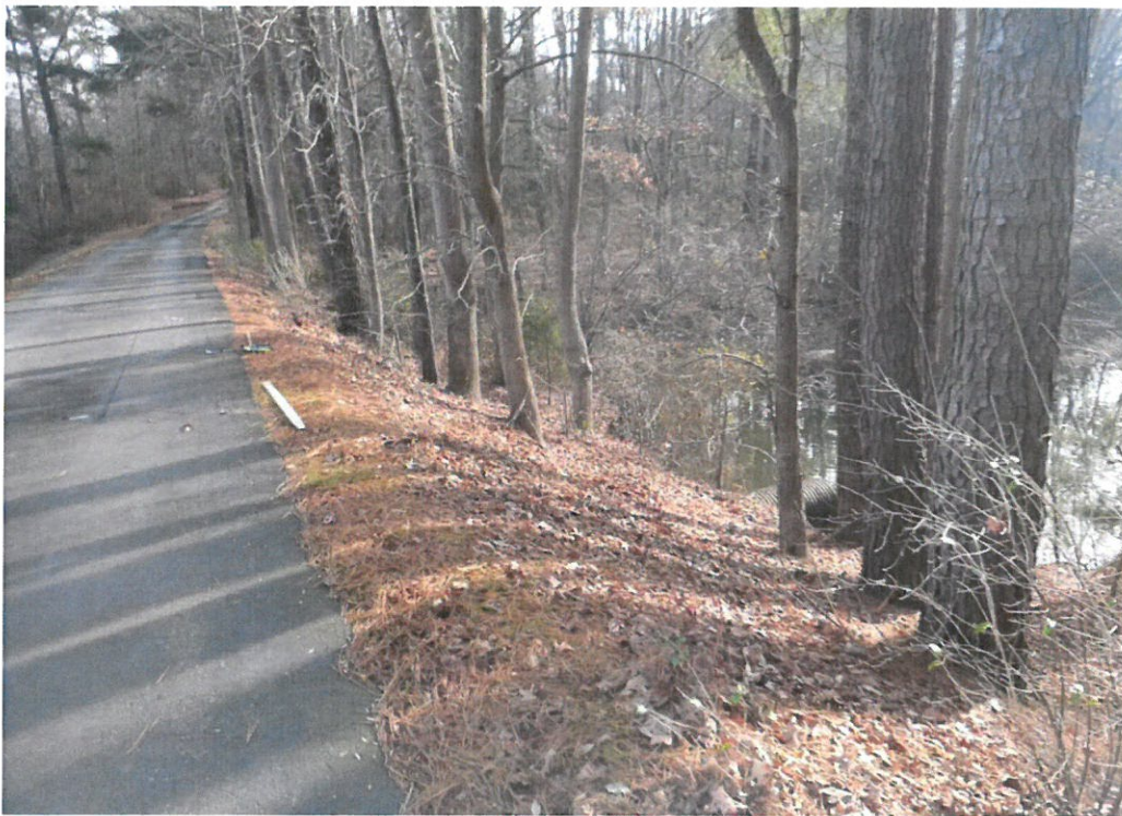
LARGE TREES ON DOWNSTREAM SIDE OF EMBANKMENT.
