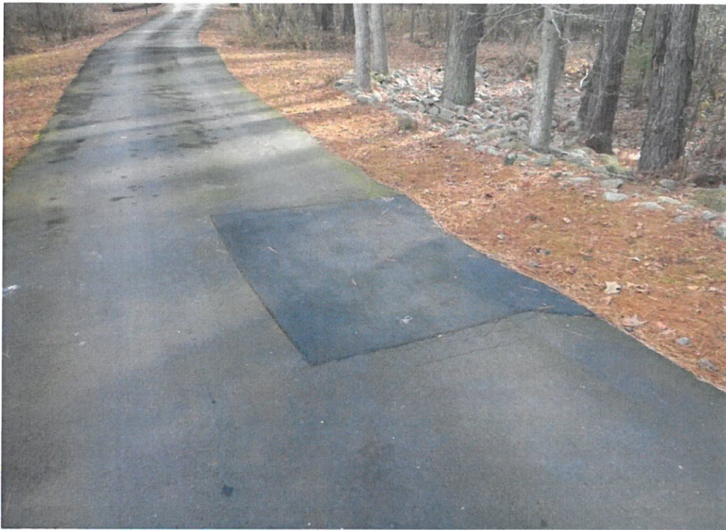
6' x 8' PATCH IN ASPHALT WEARING SURFACE INSIDE THE EMERGENCY SPILLWAY.
