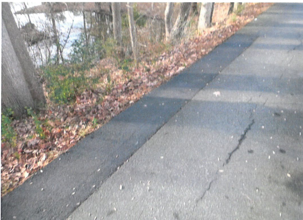
15' x 20" PATCH IN ASPHALT WEARING SURFACE ALONG SOUTH EDGE.
