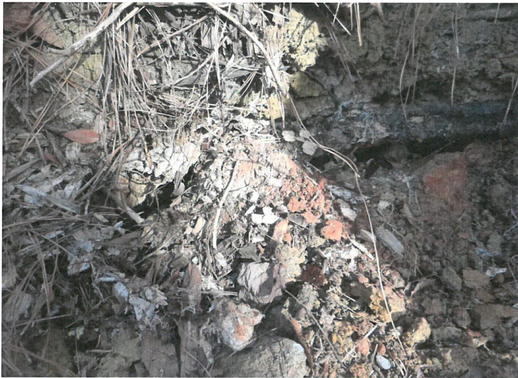
3' DIAM. X 16" DEEP SEEP ON DOWNSTREAM SLOPE.
