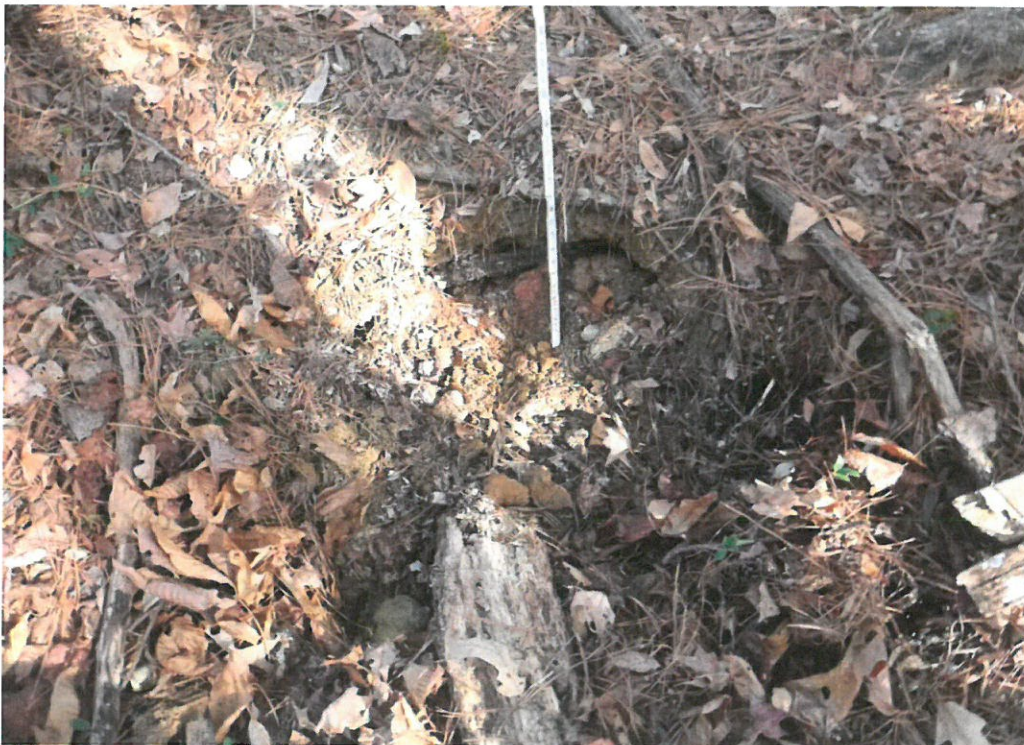
3' DIAM. X 16" DEEP SEEP ON DOWNSTREAM SLOPE.
