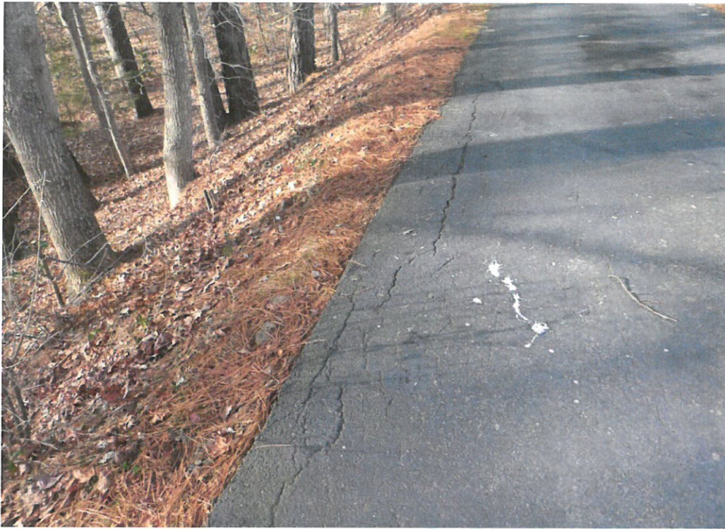
20' x 2' AREA OF SETTLEMENT AND MAP CRACKS IN ASPHALT WEARING SURFACE ALONG SOUTH EDGE.
