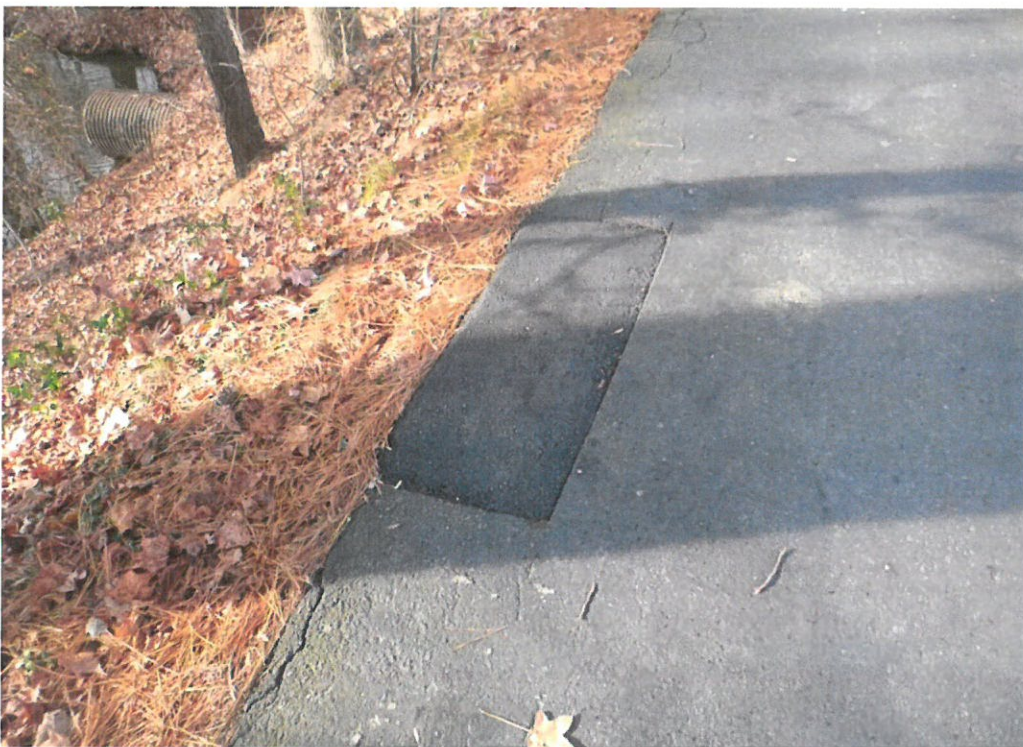
42" x 16" PATCH IN ASPHALT WEARING SURFACE ALONG SOUTH EDGE.
