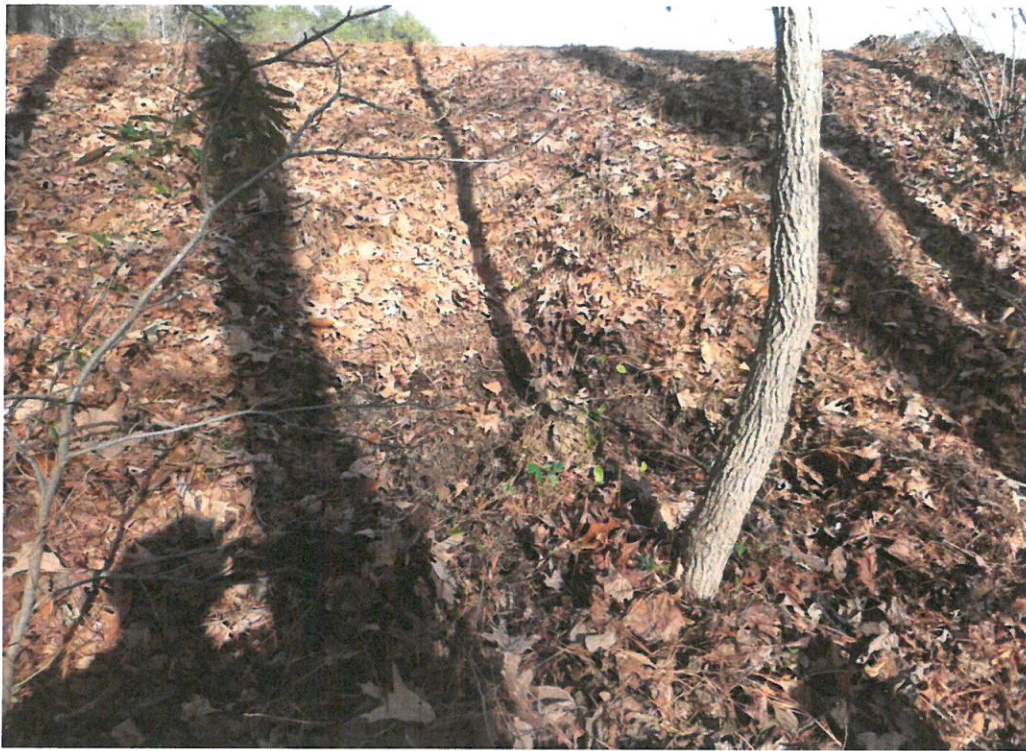
4' DIAM. AREA BY 12" DEEP SETTLEMENT AT DECAYED STUMP.
