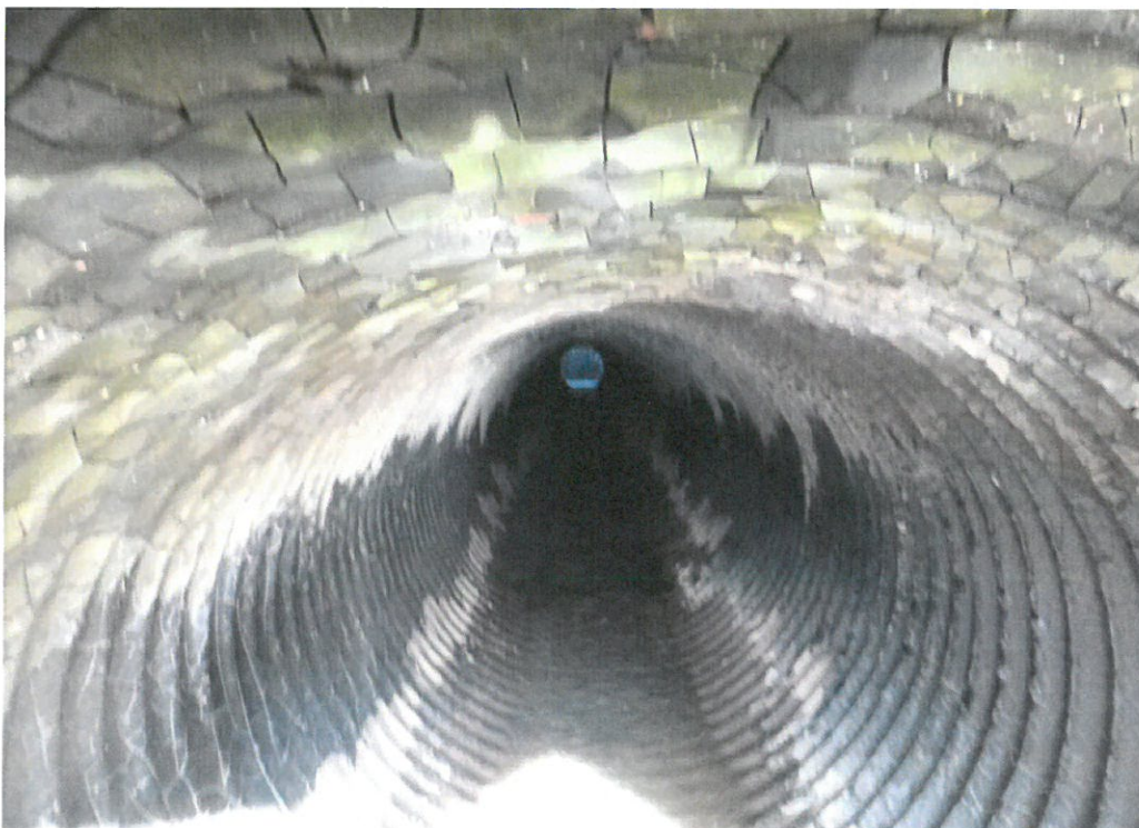
BOTTOM 2' OF COATING NEEDS REPLACEMENT INSIDE OUTLET PIPE.
